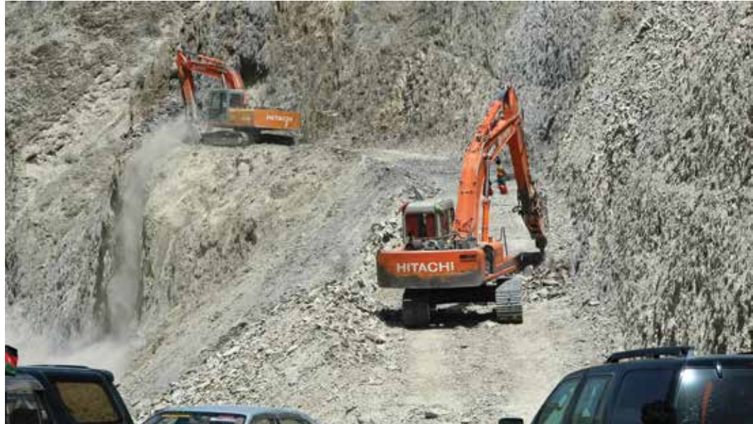
USAID road construction efforts along the Khost-Gardez road in March 2010. (USAID photo)
