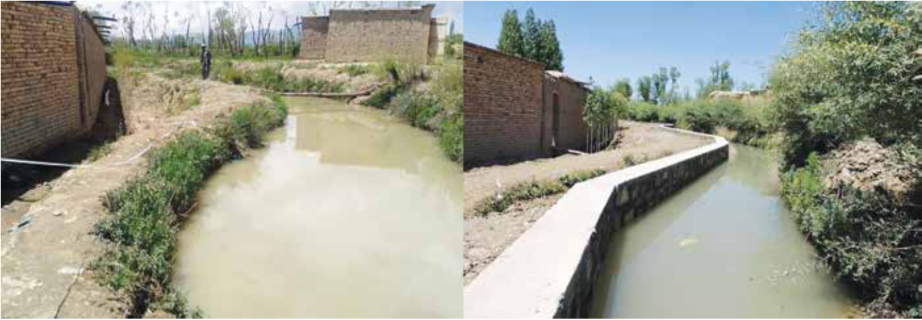
Before and after photographs of a flood protection wall built by USAID in Ahmadabad District, Paktiya Province. (USAID photo)
