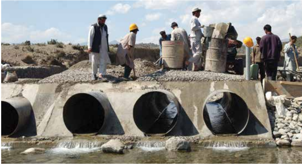
Afghan laborers build a new CERP-funded aqueduct system in Khost Province on September 23, 2006. (Photo by S. Sgt. Robert R. Ramon, 345th Mobile Public Affairs Detachment)
