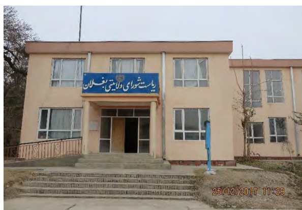
Photo 15 – Front of Provincial Council Building
