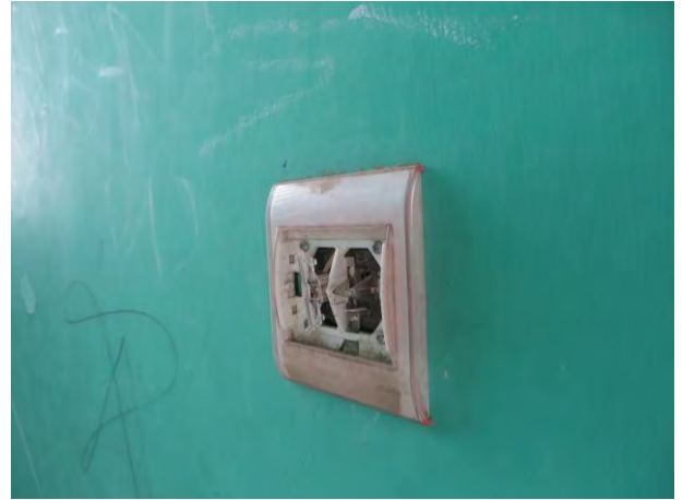
Photo 3 – Nonfunctional wiring to lights and sockets at School S229A in Kunduz City
