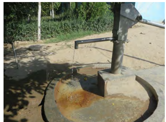
Photo 5 - Functioning Well at School S229A in Kunduz City
