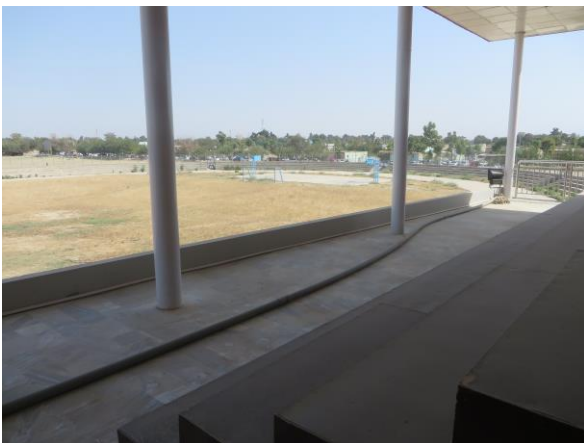
Photo 3 – Unused Track, Football Field, and Basketball Court at Kunduz Stadium
