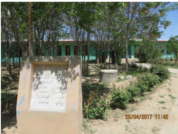
Photo 2 – Empty Facilities at School SR 168
