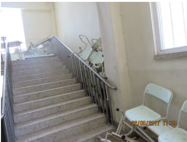
Photo 10 - Broken furniture pile at School KSP001
