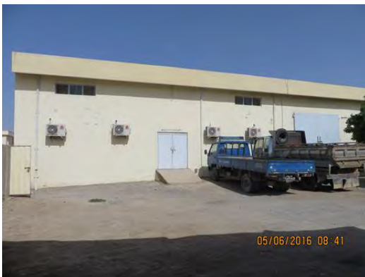
Photo 1 – Front of Storage Facility
