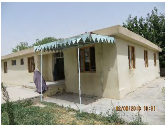
Photo 5 – Front of Facility 747
