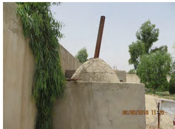
Photo 8 - Incinerator at Facility 747
