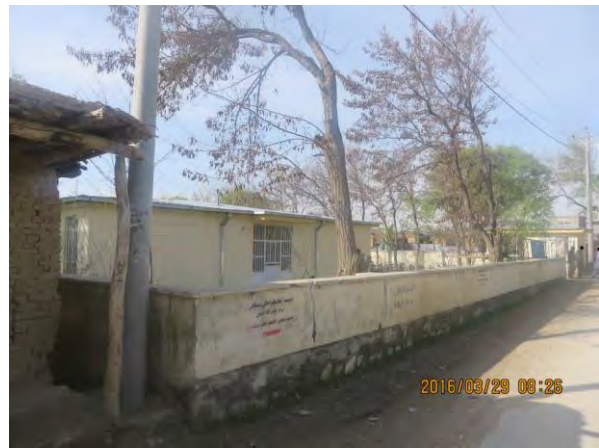
Photo 3 – Power Lines Outside School SKP-3 in Hisa e Awal Kohistan
