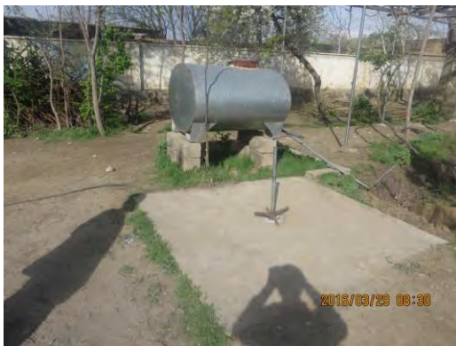
Photo 4 - Broken Well Pump at SKP-3 in Hisa e Awal Kohistan
