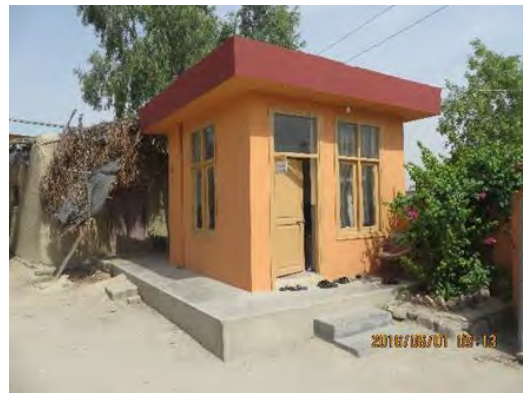
Photo 6 – Guard House Health Facility 1214
