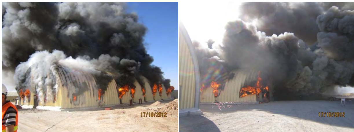
Figures 1 and 2– Fire at Classroom building 906 at Afghan National Army Brigade Camp Saher near Farah Province, Afghanistan on October 17, 2012. Source: US Army Corps of Engineers. The fire incident report noted the building was 85 percent completed and burned in 30 minutes.
