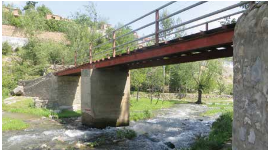
CERP-funded pedestrian bridge in Kabul. (SIGAR photo)
