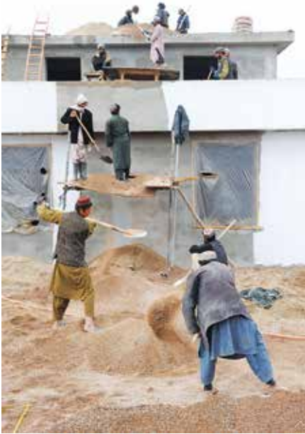
Workers move gravel up to the roof of a new prison in Uruzgan Province, 2011. (USAF photo by 1st Lt. Matt Schroff)
