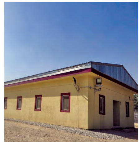
Newly constructed barracks at Camp Commando, Kabul. (SIGAR photo)
