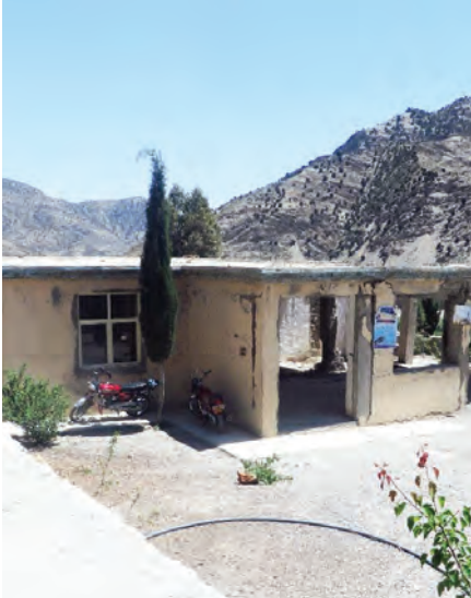
USAID support benefits a health facility in Khowst Province via the World Bank-administered SEHAT program. (SIGAR photo)
