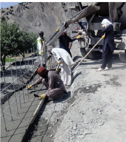
Workers install concrete for a highway project in southeast Afghanistan. (USAID photo)
