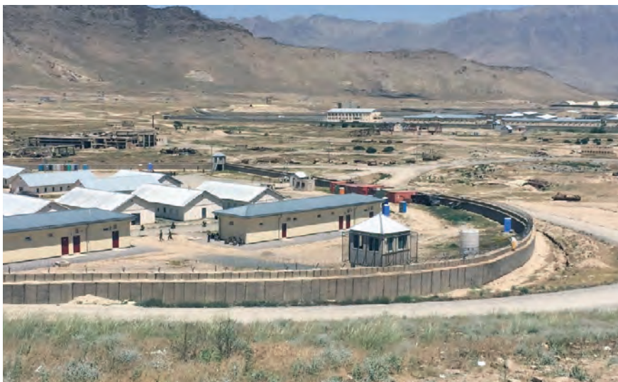
Kabul Military Training Center Phase 4 Forward Operating Base area (Photo by CSTC-A CJ-Eng)
