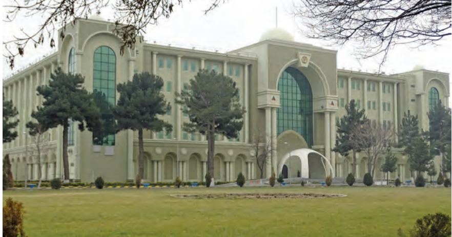
Afghan Ministry of Defense headquarters building in Kabul, January 7, 2016. (SIGAR photo by Wilhelmina Pierce)
