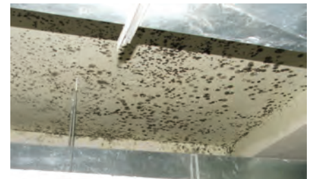
Mold growth in bathroom at Afghan Air Force University, March 2015. (SIGAR photo by Javed Khairandish)
