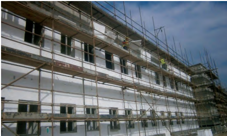
Construction of the Marshal Fahim National Defense University Joint Service Academy building in Kabul. (CSTC-A photo)
