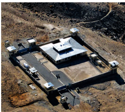
This Afghan National Police district headquarters in northern Afghanistan is one of many facilities built under contracts awarded by the U.S. Army Corps of Engineers. SIGAR has found some ANP facilities to be under- or unutilized. (USACE photo)
