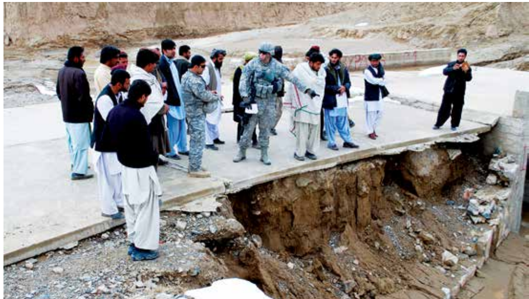
U.S. Air Force Tech. Sgt. Latha Caillouette, a PRT Zabul engineer, shows contractors erosion control repairs that are needed at a bridge in Shah Joy District, Zabul Province, on March 4, 2011. (U.S. Air Force photo by 1st Lt. Brian Wagner)
