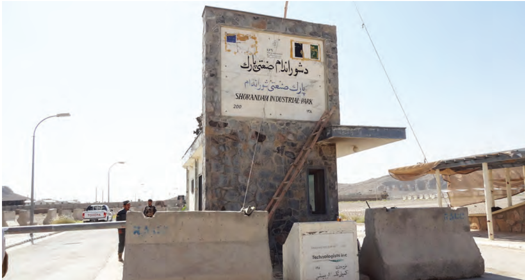
Main entrance to Shorandam Industrial Park in Kandahar in June 2014. (SIGAR photo)
