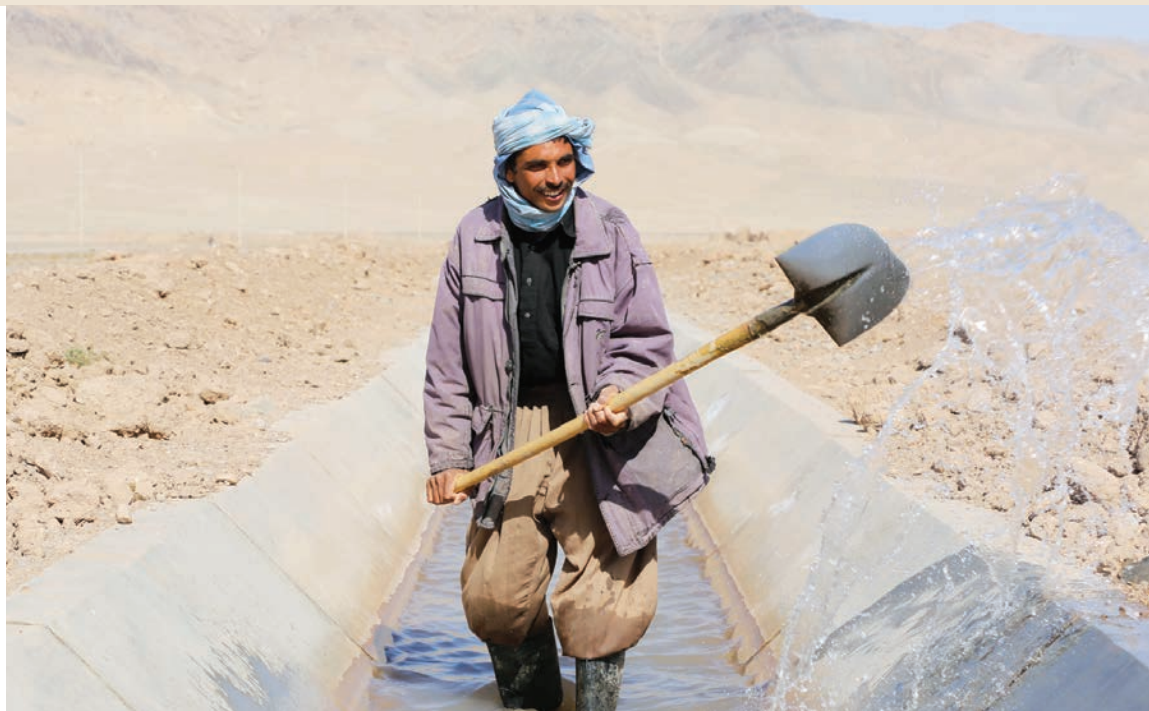
Afghan farmer clears silt from a newly cemented irrigation ditch in Herat Province. (World Bank photo)
