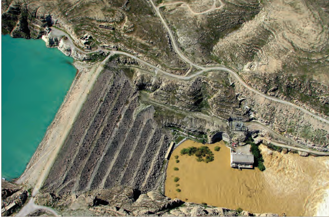
An aerial view of the Kajaki Dam in Helmand Province, a key part of the Kandahar Helmand Power Project. (USAID photo)
