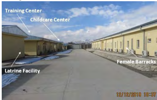
Photo 1 - Facilities Constructed at the Afghan National Police Women's Compound at the Gardez Regional Training Center
