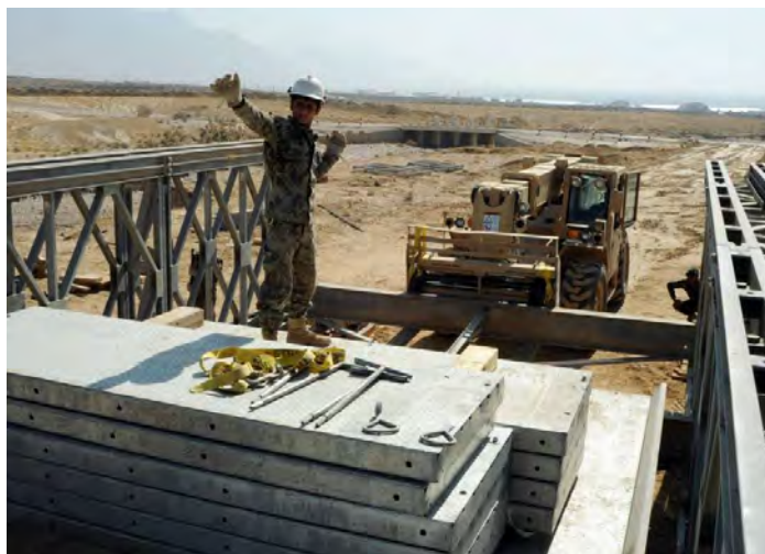
Photo 1 - NEB Portable Bridge Training Exercise
