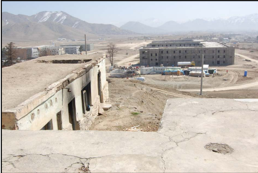
Photo 1: ANSU Construction Site
