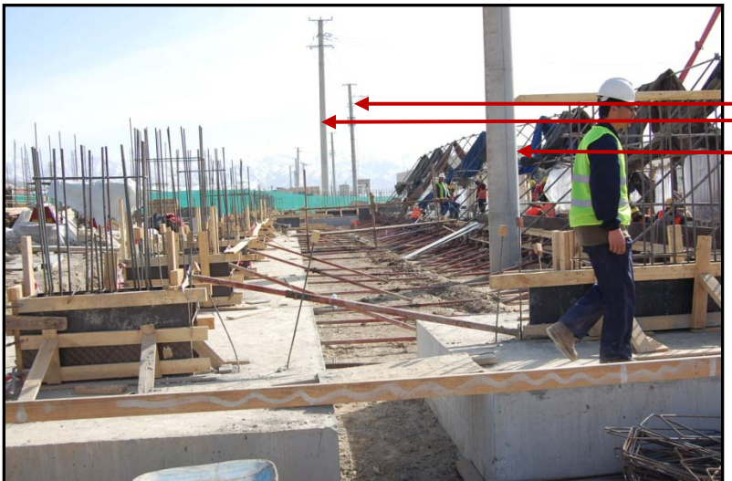
Photo 4: KMTCC Phase III Construction Site
