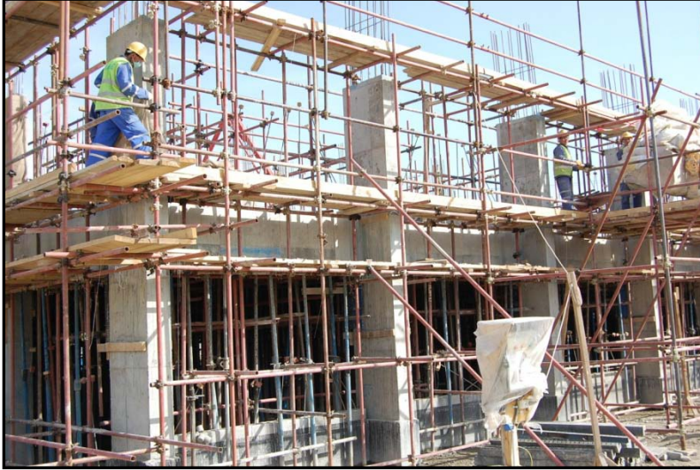
Photo 2: KMTC Phase III Ongoing Construction
