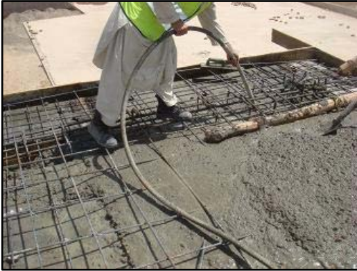
Photo 2: Placement of Watery Concrete Mix
