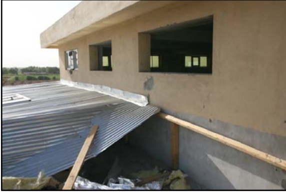
Photo 9: Partially Demolished Roof at Nad Ali Site
