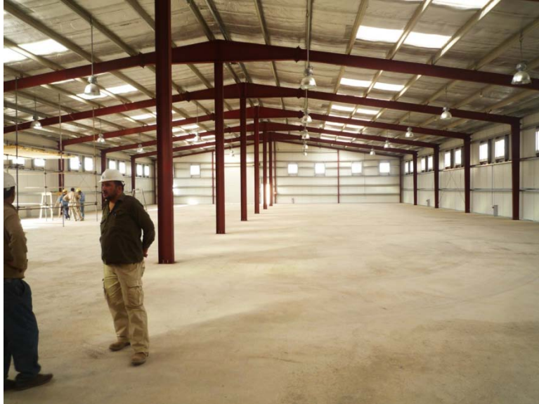
Photo 1: Interior View of the RLC Warehouse
