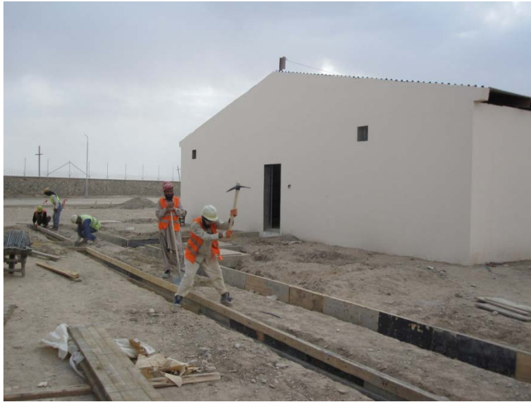
Photo 7: Construction Outside BP Barracks
