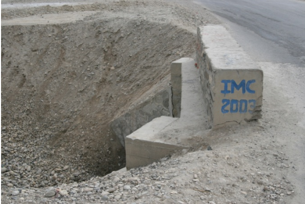
Photo 5: Bridge Near Entrance of the Gamberi ANA Garrison
