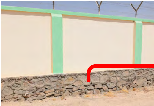
Photo 10 - Boundary Wall and Foundation
