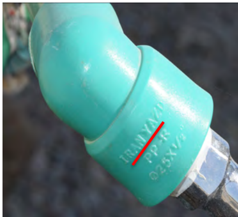
Photo 2 - Prohibited Piping from YAZD Pipe
