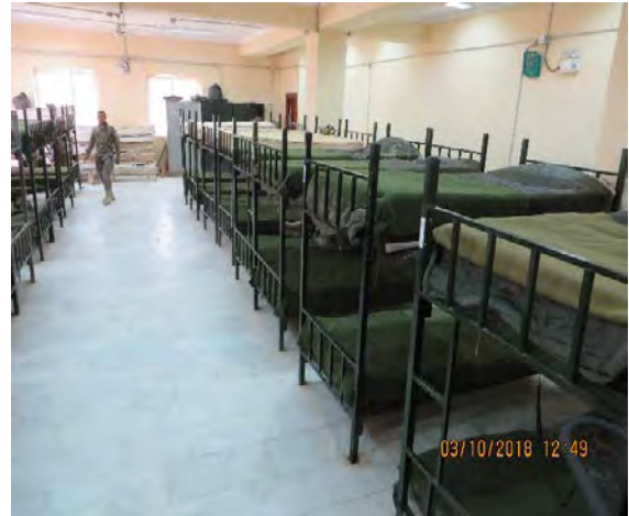
Photo 7 - Renovated Building 404 Used as Barrack Instead of Training Classroom Building
