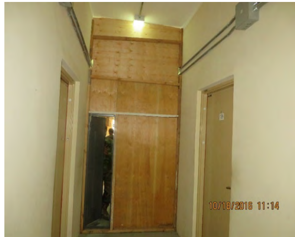
Photo 9 - Permanent Wooden Wall Blocking Main Corridor of Noncommissioned Officers' Barrack 603
