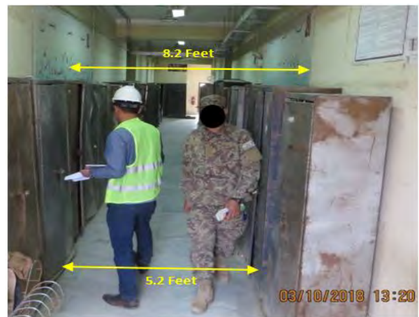
Photo 8 - Lockers on Both Sides of Corridor Walls in Renovated Classroom Building 402
