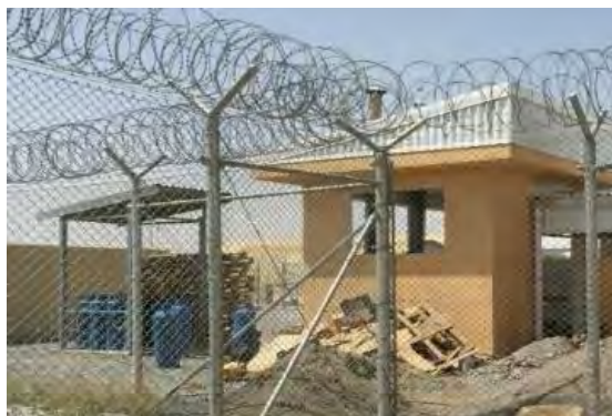
Photo 3 - Propane Tanks Stored Too Close to the Cooking Building
