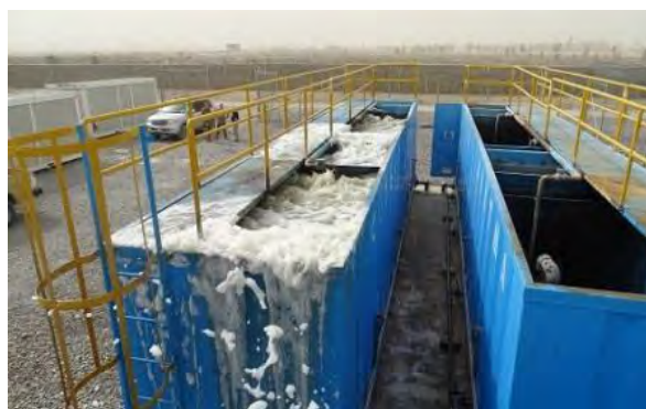
Photo 2 - Wastewater Treatment Plant with One Functioning Tank
