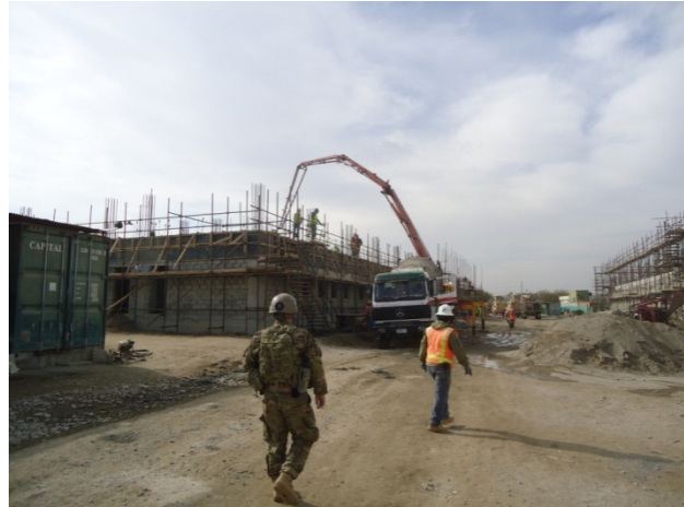
Figure 7 - Roof Slab Pour Underway for Administration Building
