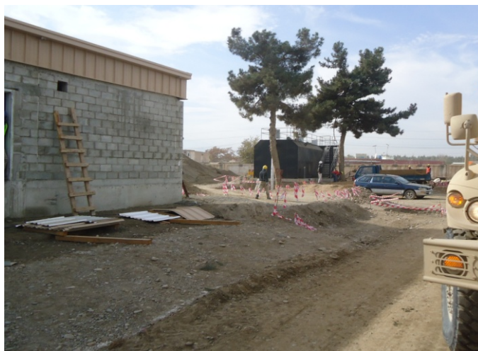
Figure 8 - Distant View of the Sewage Treatment Plant
