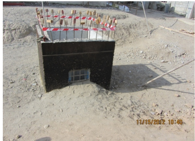
Figure 3 - Sewer Manhole Construction
