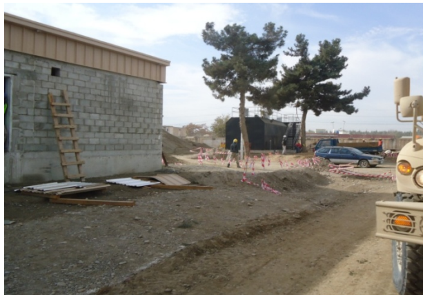
Sewage Treatment Plant (black) at Elevated Portion of Provincial Police Headquarters Compound
