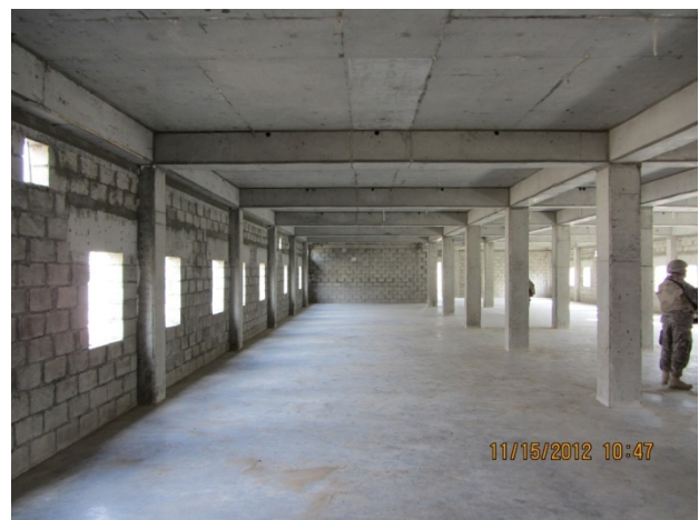
Figure 5 - Open-Bay Barracks under Construction
