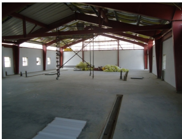
Figure 4 - Dining Facility under Construction
