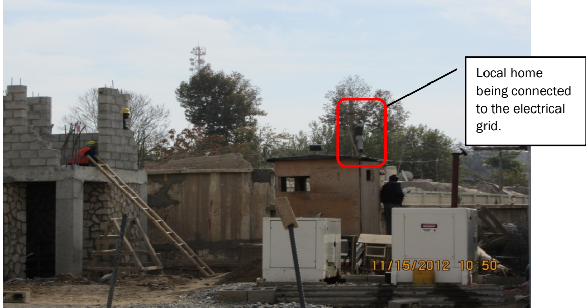
Figure 11 - Evidence of Local Electrical Grid Adjacent to Site
