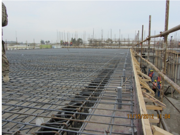
Figure 6 - Roof Rebar Placement for Concrete Pour for Open Bay Barracks
