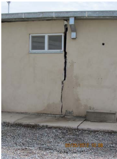
Figure 7 - Exterior of Building 603
