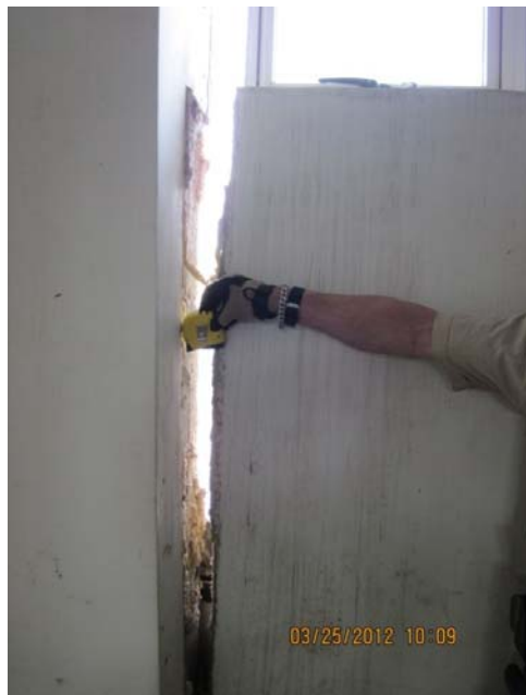
Figure 6 - Interior of Building 603
