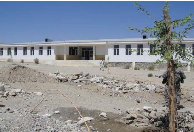
Site Photos 5 and 6: Views of the school yard that the Kohi Girls' School shares with the adjacent boys' school (left). SIGAR believes that the statement of work should have included removal of such hazards. (Photos provided by SIGAR)
