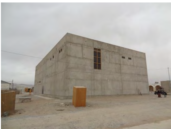
Photo 1 - Exterior of Building
