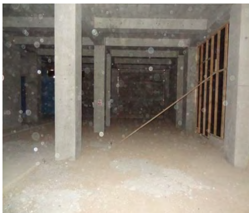
Photo 2 - Interior of Building
